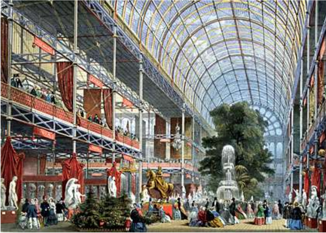
Crystal Palace with intricate iron framework and curved glass (all modular). This elm tree at transept was among a few more.
