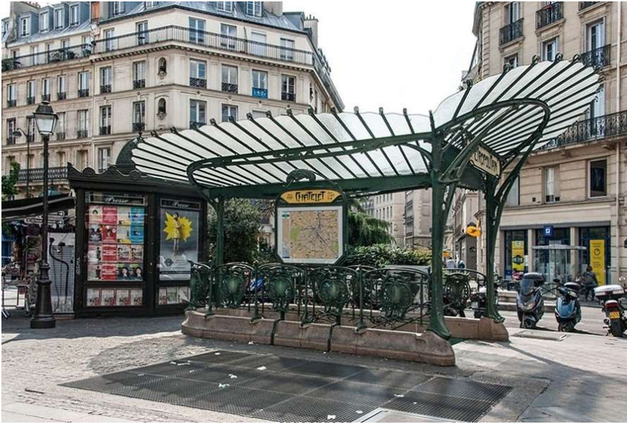
3 One of the Paris Métro gates designed by Hector Guimard with cast iron, glass canopy, and floral motifs. Collection: Flickr user Alain Roy
